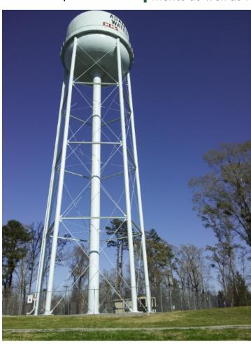
County Board of Supervisors selected JKS to perform the engineering design and construction management services associated with the CCA project which involved the installation of a 1.200 feet deep, 1,000 gallon per minutes well, and disinfection controls building, a 350,000 gallon tank and approximately one mile of 10" PVC water main. . The total construction cost of the project was funded through the CDBG Program. This system is operated by Adams County Water Association.
